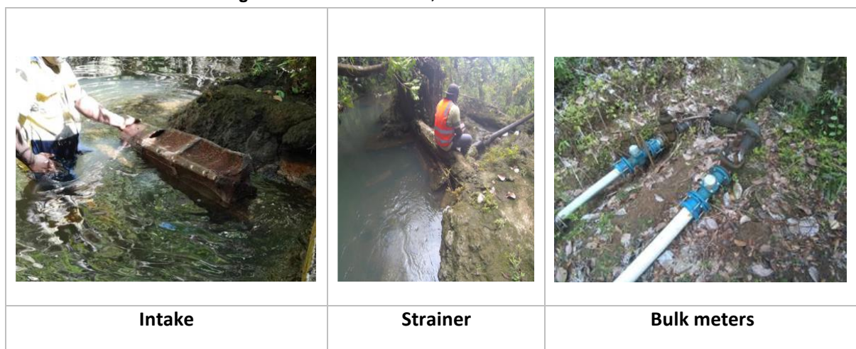
Figure 1-3: Maleali Intake, Strainer and Bulk meters
