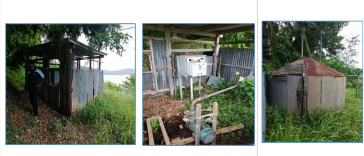
Figure 1-4: Photograph of Pumping Station and 0.015 ML Suction Tank in Tulagi
