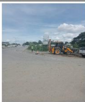
1. Missing barricades and appropriate speed limits signages.
