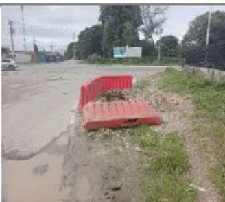
4. Broken water filled barriers knocked over by wind and rain. 5. No sediment control in place.
