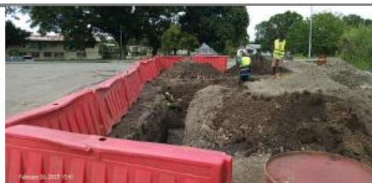
11. Broken water filled barriers continue to be used in eastern section at Burns creek site.
