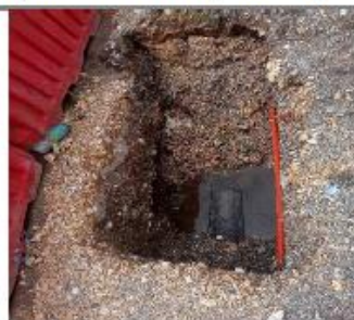
6. Open pit increases likelihood of sediment buildup in pipes, added risk to public safety and moving vehicles.
