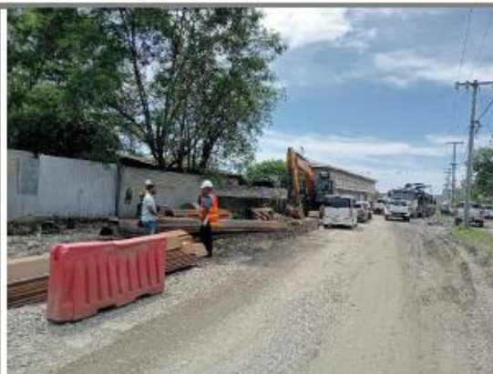
Poor traffic management leads to traffic congestions and increase dust concentrations on site. There is also no portable toilet available for workers.
