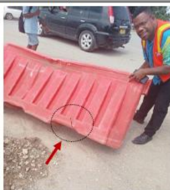
2. Broken water filled barriers consistently used in project sites.
