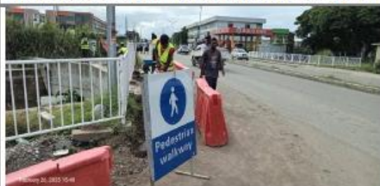
10. Improper pedestrian walkway, no cones and tapes.
