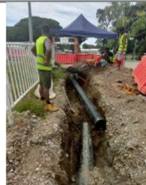
3. Workers exposed to incoming traffic with inadequate barriers.
