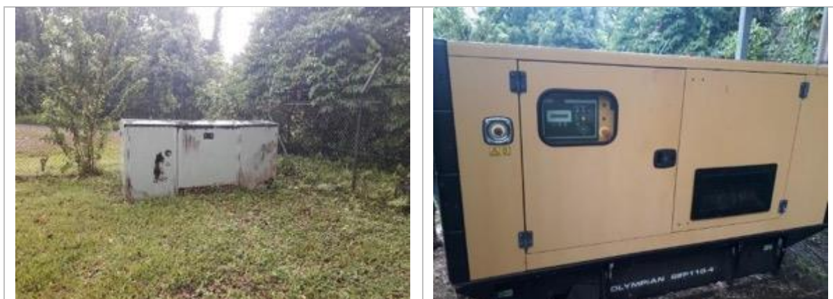
Plate 4-10: Transformer, Generator Set (110 kVA) and Electrical Cabinet
